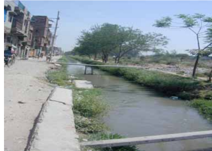
Unlined open drains – source for groundwater pollution
